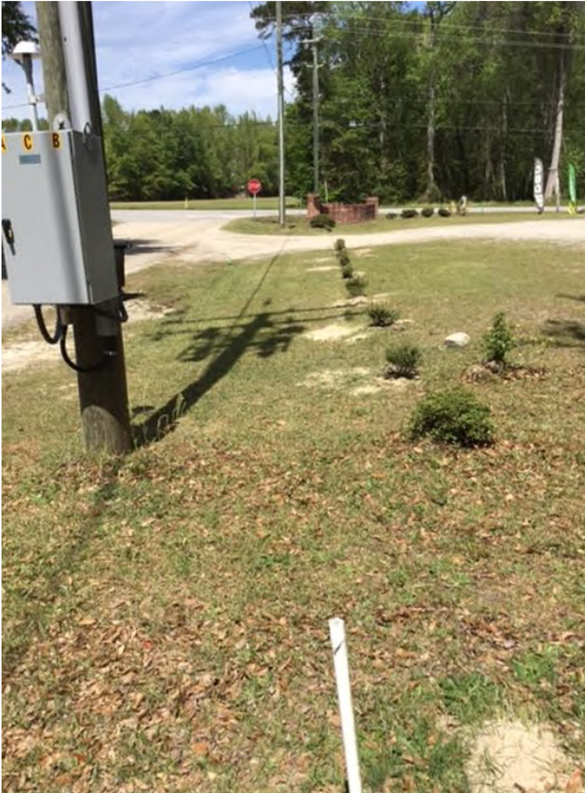
Inadequate landscaping and unapproved driveway access along Elgin Estates Drive
