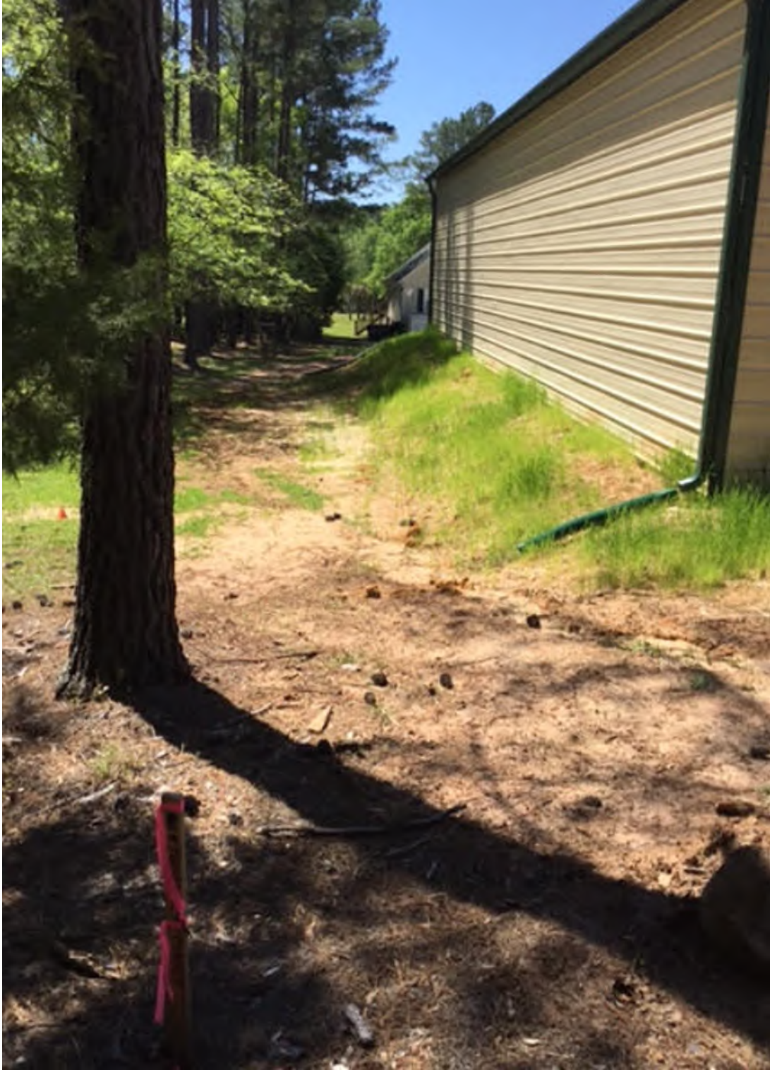
View of left side of Accessory Building from Darby Road
